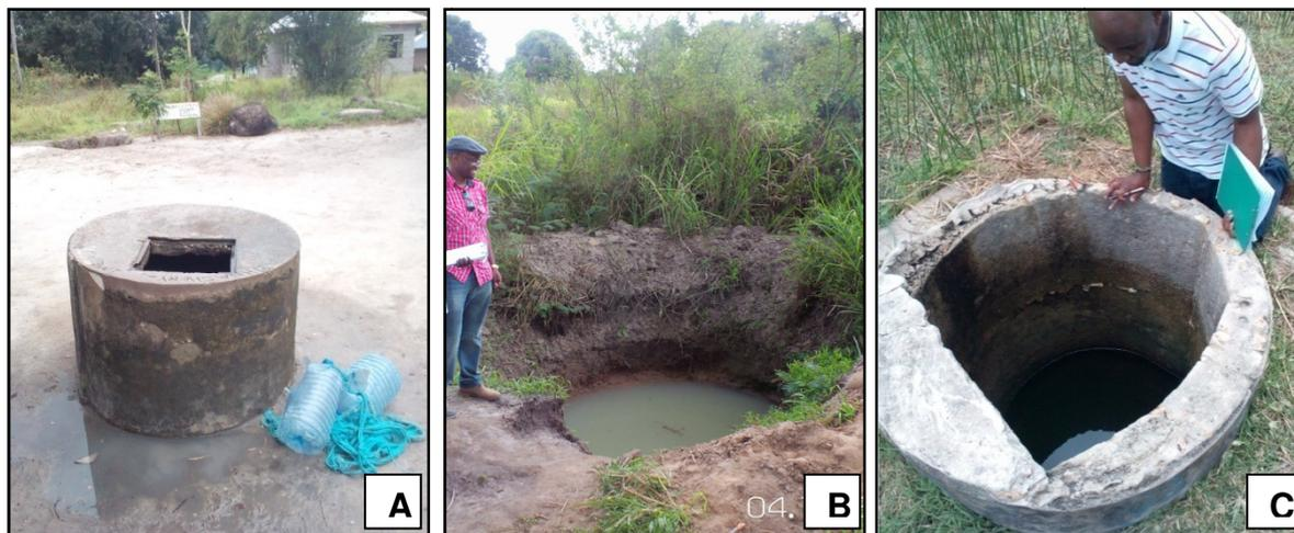
Figure 5-10: Examples of unimproved water sources, unprotected deep well (A), a hand-dug shallow well (B), and open shallow well (C) as found in Kiromo and Zinga wards (October, 2014).
