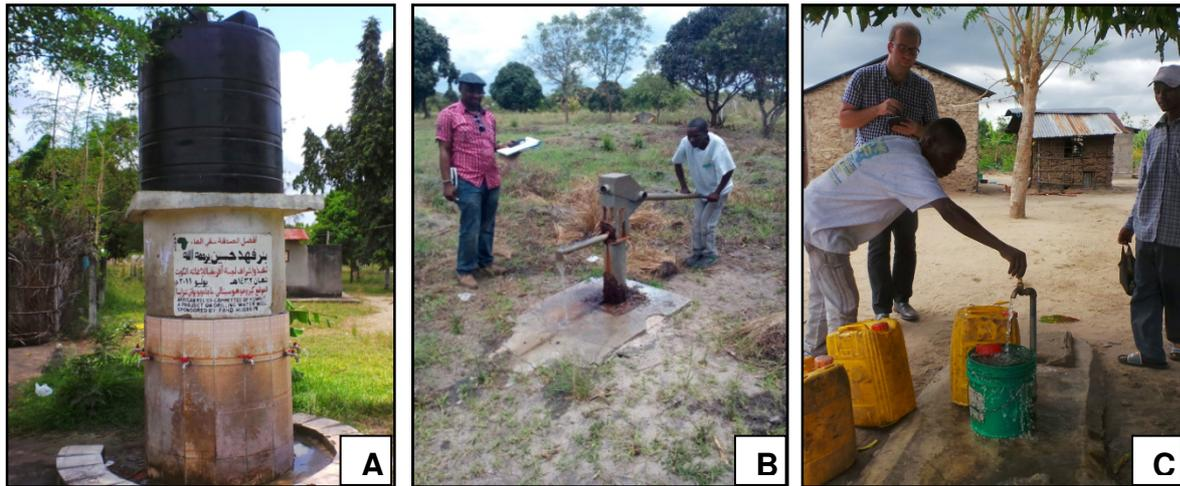
Figure 5-9: Examples of common types of improved water source, a borehole (A), a hand pump (B), and a standpipe (C) as found in Kiromo and Zinga wards (October, 2014).
