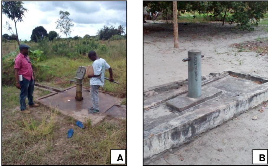
Figure 5-3: Examples of functional (A) and non-functional (B) public water points as found during mapping in Kiromo and Mandawe sub-villages (October, 2014).
