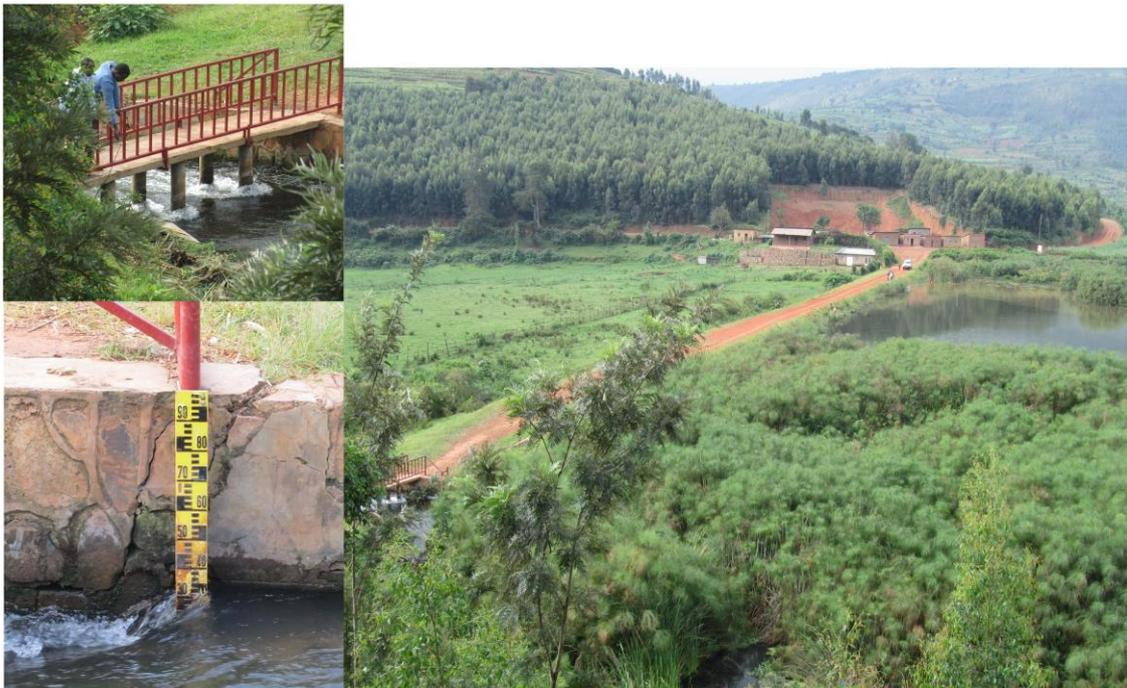
Figure 4-11: Lake Muhazi outlet dyke (top left), lake gauging scale (bottom left) and vegetation covering the outlet of the lake (right).
