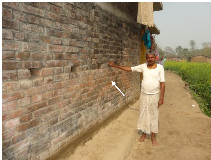
Figure 4.8 Flood level marks on the wall
