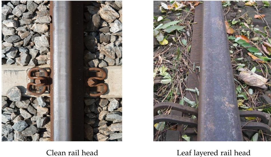
Figure 2.4: The left picture is a clean rail head and the right picture is a leaf layered rail head(ProRail, 2020)
