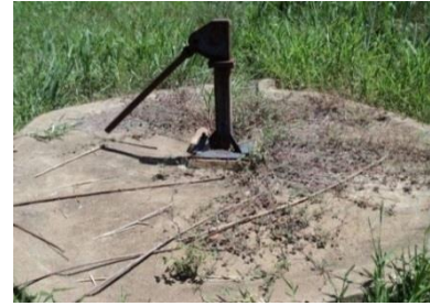
Non-functional SWN 80 water point from Mvuha ward in Dala village at Morogoro rural district.
