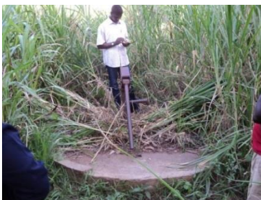
Non Functional Water Point (SWN 80) found around the bushes at Kiroka Ward in Kikundi village in Morogoro rural district.
