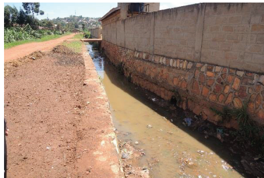
This was presumably the longest and widest drainage channel cutting across the study area. This photo was taken at location Point 11 , with a width measurement of 3.8 m and a depth of 6m. This measurements however varied at various points/locations of the channel
