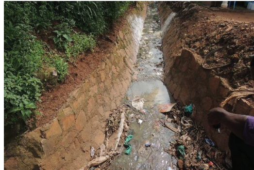
Drainage channel passing through Masanafu village- Spatial location is shown by Point 22 on the map. Although the drainage channel was fairly big, parts of it were had garbage deposits that definitely hindered the smooth flow of waste water
