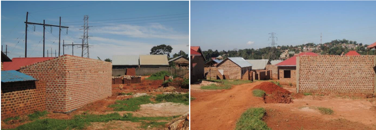
Figure 5.3: New Developments (Infilling) in the study area Source: Field Survey, 2013
