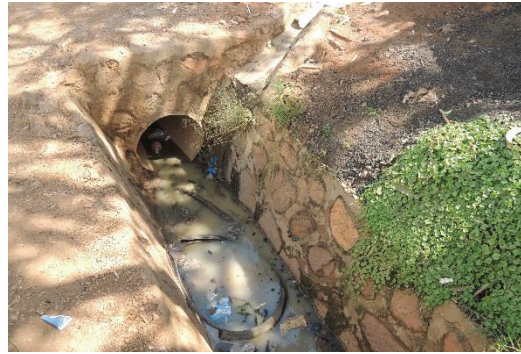
Point 21 -Drainage channel located in Lugala Village. The width of the channel measured approximately 168 cm.
