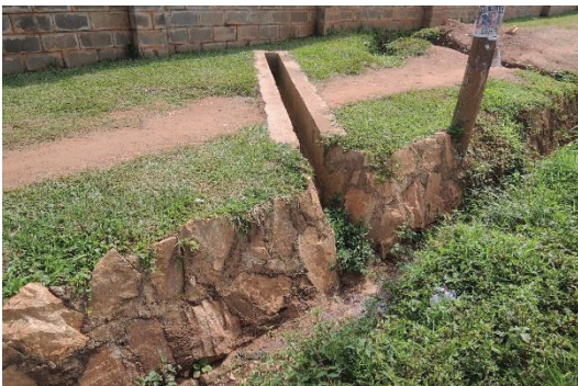
Smaller Drainage Channels connecting at plot level at point 20 in Lubia village
