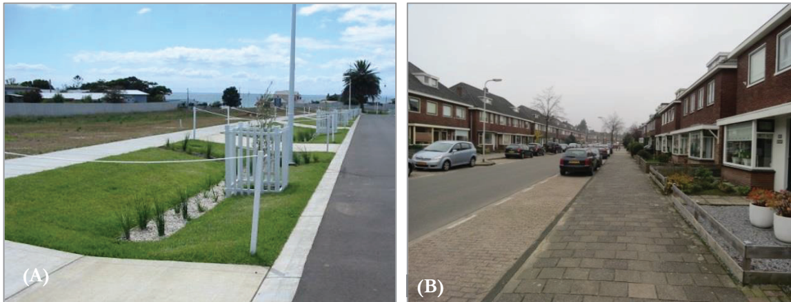
Figure 5-11. Vegetated swales (A) Example of the vegetated swales. Source (Water Sensitive Urban Design in Sydney, 2014). (B) Potential site for this measure, Elferinksweg street. (Photograph by author).
