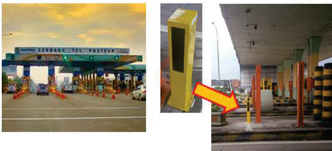
Figure 8 Optical beam detector at each of toll booth at Pasteur toll plaza
