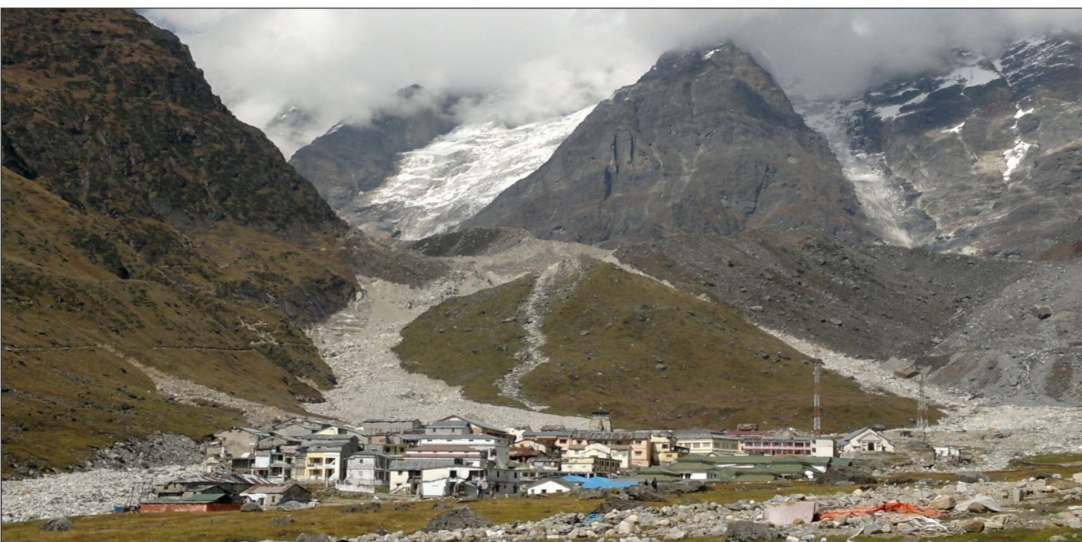
Kedarnath township after the disaster (field photos, dated October 17, 2013)
