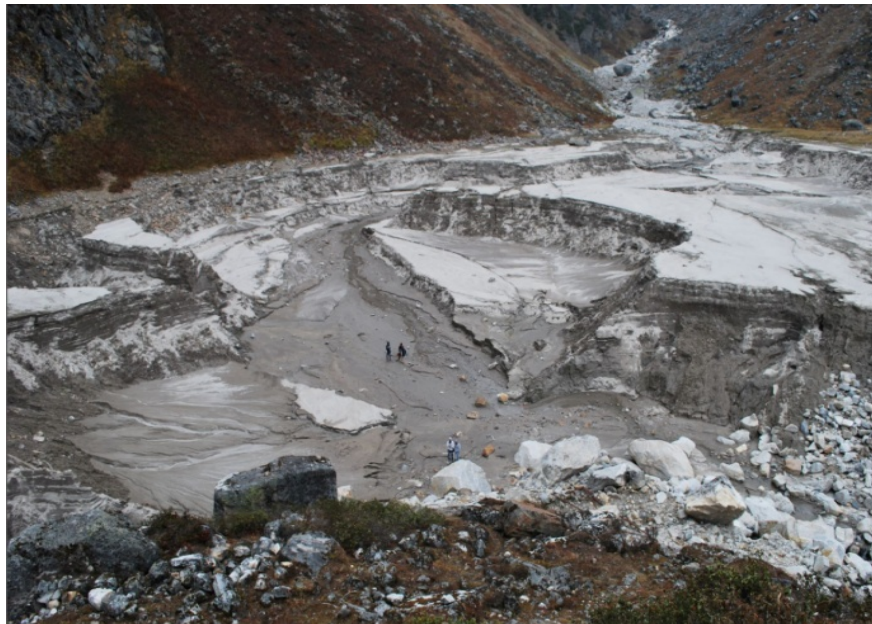
Figure 2: Chorabari lake after disaster (Field photograph)
