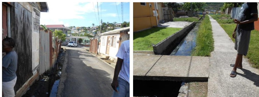
Figure 6-6: Drains filled with silt
