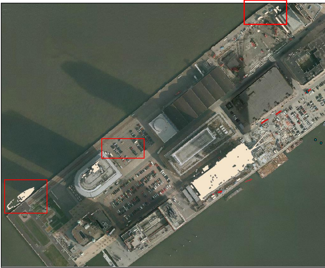
Figure 4-13: Aerial image showing the ground truth of false positives in buildings in 2010 as in figure 4-12
