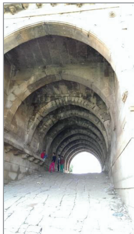
Photo 7: Outlet gate to river
