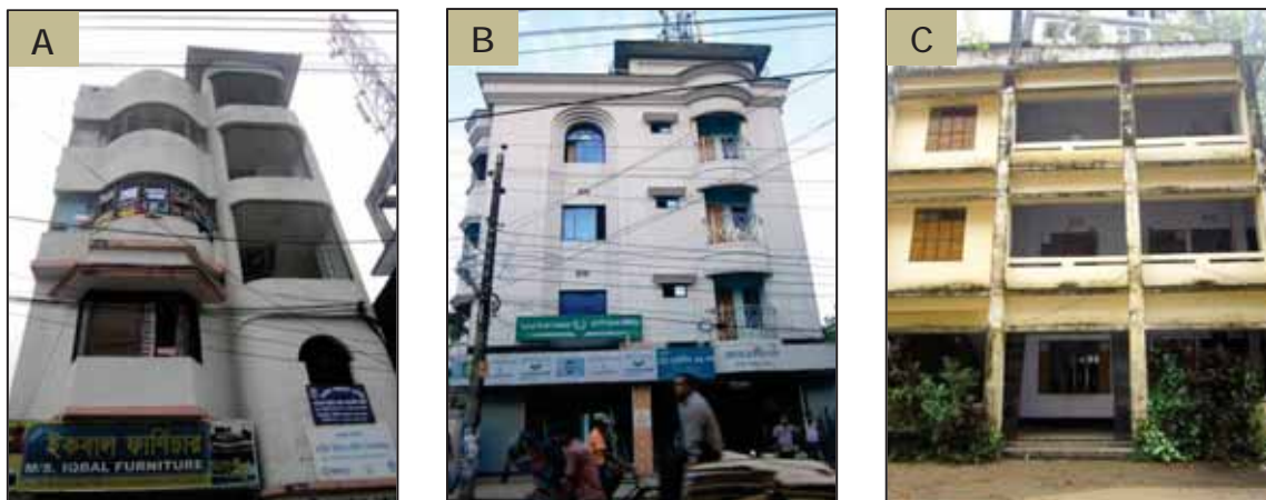
Figure 5-3: Structural type misclassification: A & B (mixed-use building) classified as BFL building; C (a school) classified as C4M instead of C4L
