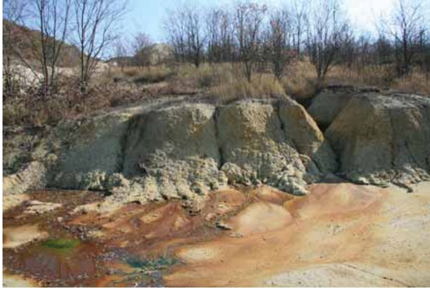
FIGURE 3.10: Seepage of Acid Mine Drainage (AMD) at the base of tailings dam 1 (Krivelj TDF1). The AMD is the result from pyrite oxidation as given in equation 2.2. This gives rise to the formation of Goethite/Hematite that inhibits the typical brown/red staining of the seepage water. [1st November 2011, Bor, Serbia (44°5'58.3" N; 22°7'48.8" E)]
