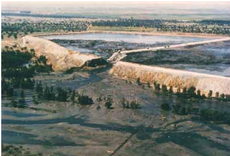
FIGURE 3.1: Failure of the Los Freiles tailings dam, releasing approximately 6.8 million m 3 tailings into the surrounding. The accident took place on 25th April 1998 in Aznalcóllar (Andalusia, Spain). [Alonso et al (2010) 22 ]
