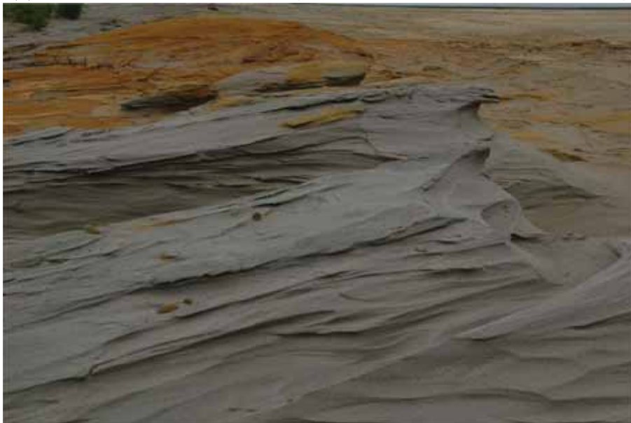
(B) Wind erosion on the crest of the tailings dam. [5th March 2011 (44°5'12.3" N; 22°9'35.8" E)]
