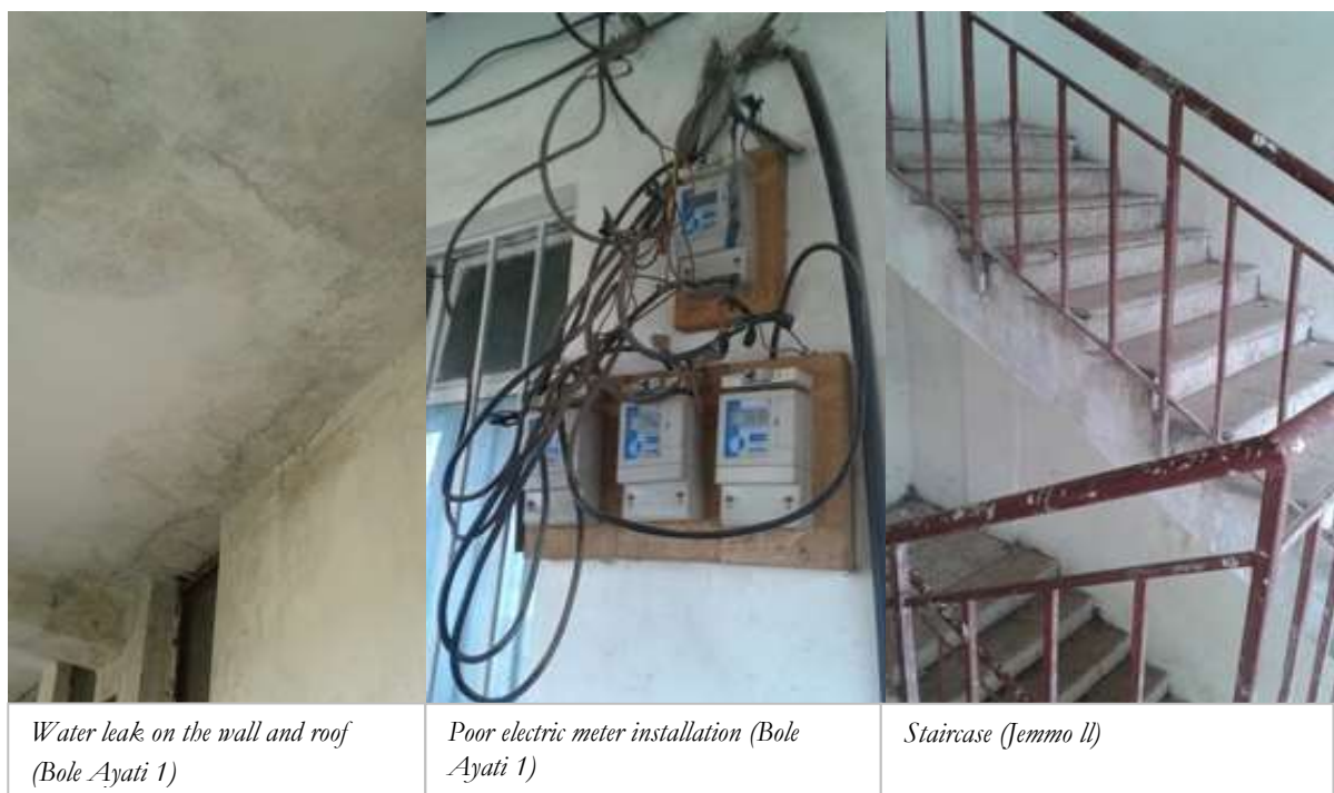
Figure 5.10 Structural quality problem in urban periphery condominium sites
