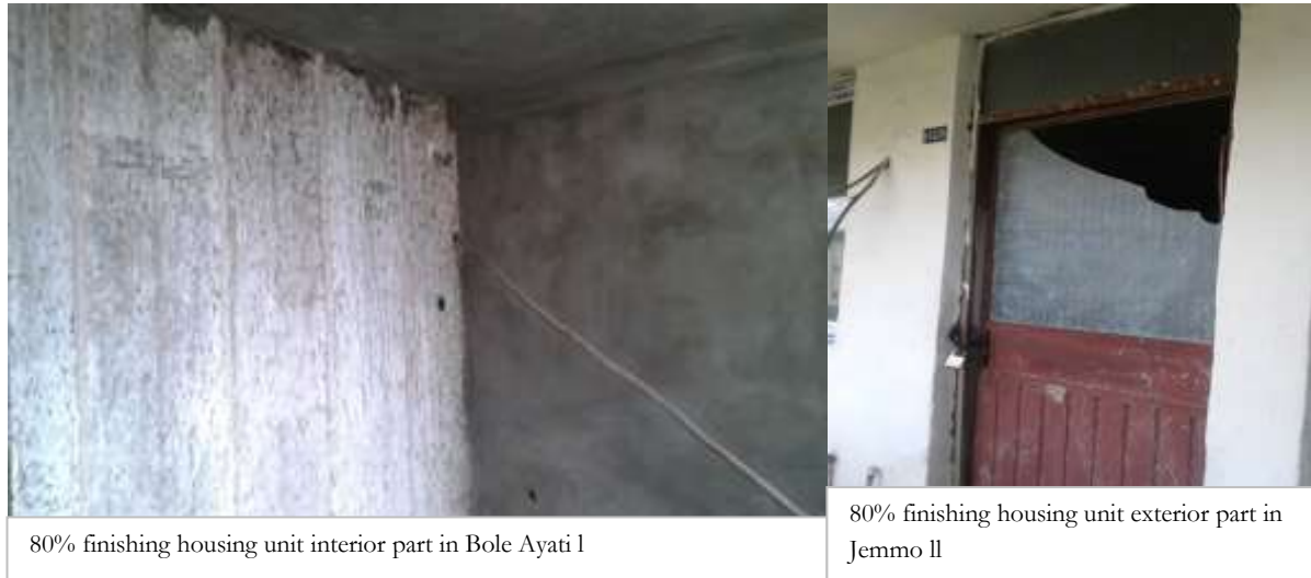
Figure 5.12 Condominium housing unit finishing stage
