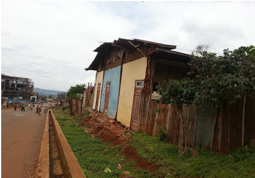
Figure 5-6: Picture of Partially Demolished Residential House in the Study Area
