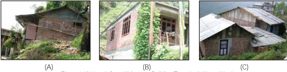
Figure 4-13 Un-reinforced Masonry Building Types in Arithang Ward
