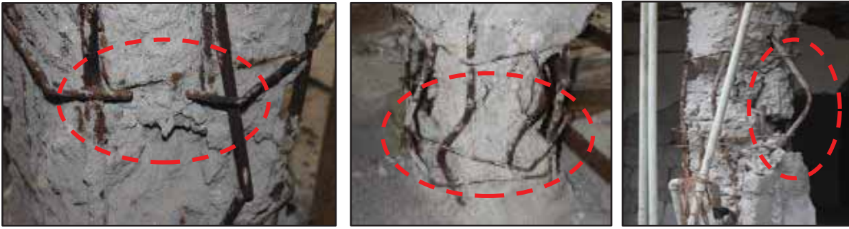
Figure 5-18 Reinforcement failures
