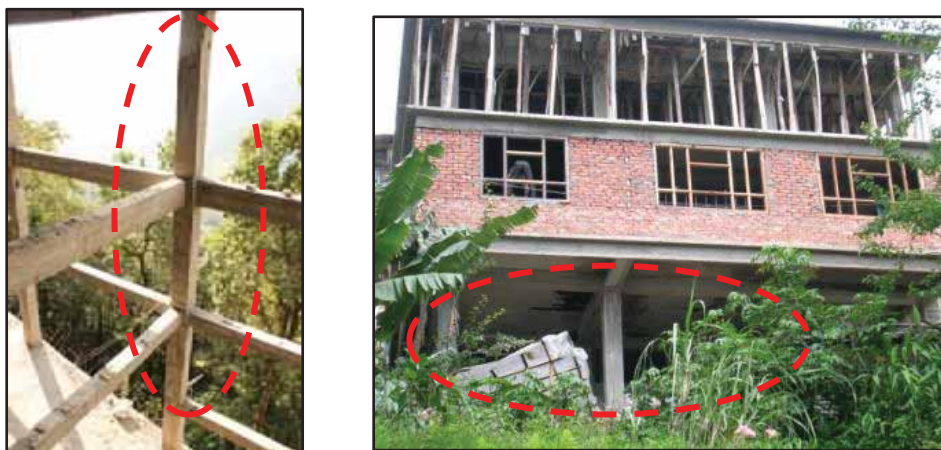
Figure 5-20 Absence of shear walls
