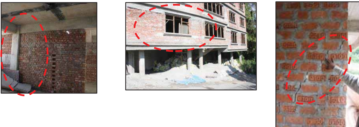
Figure 5-15 Unreinforced Masonry infill's
