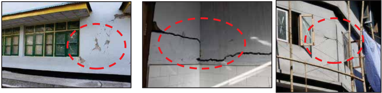
Figure 5-16 Damages in Unreinforced Masonry infill's
