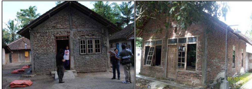
Figure 41 Example of building structure RM2L in Peni Sub-village
