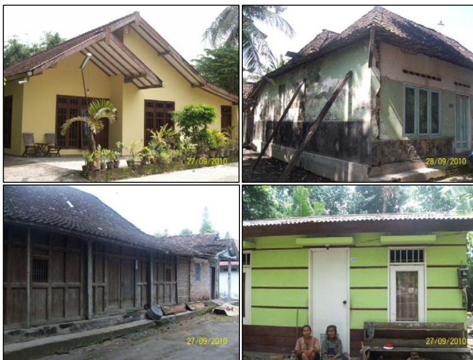
Figure 19 Building types in study ward area in Palbapang Village, Bantul. RM2L type (top left), URML type (top right), S1L type (down right) and Wood type, W1 (down left)
