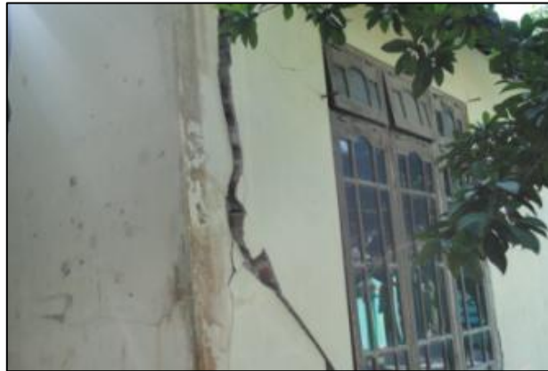
Figure 36 Example of building structure URML in Bolon Sub-village
