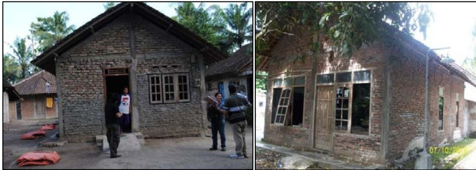
Figure 39 Example of building structure RM2L in Peni Sub-village
