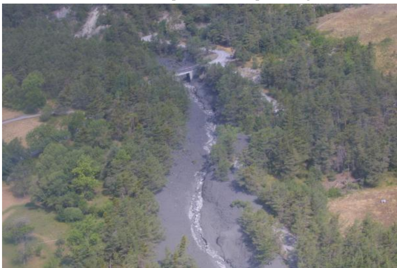
Debris flow deposits at the Apex Bridge
