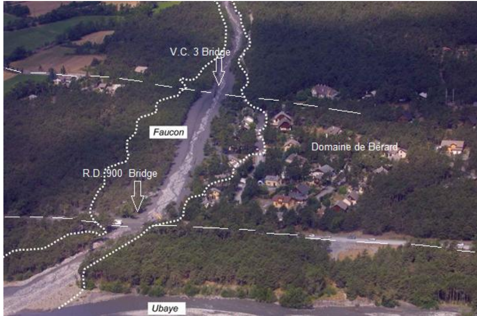
Figure 15 The 2003 debris flow run-out affecting Domaine de Bérard and blocking two main bridges (adapted from: Remaître (2006))
