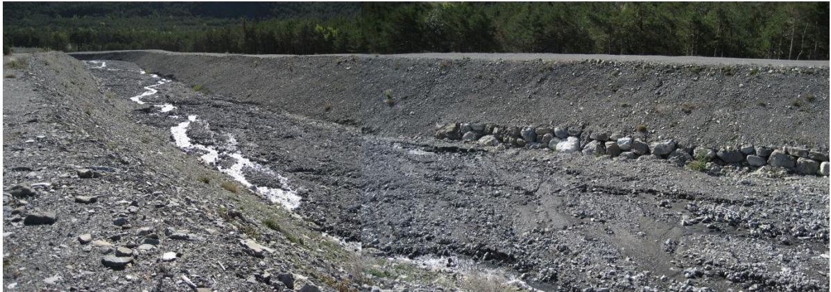
Figure 10 The Faucon torrent and its dikes at the debris fan (1202 m). It is managed by the French Forestry Office (ONF)
