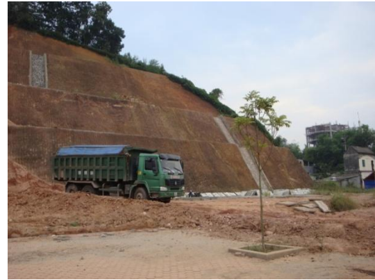
Figure 6-7: Application of benching method in Hoa Binh street, Yen Bai
