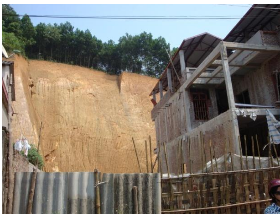
Figure 1-1: Slope cuts to create space in Yen Bai
