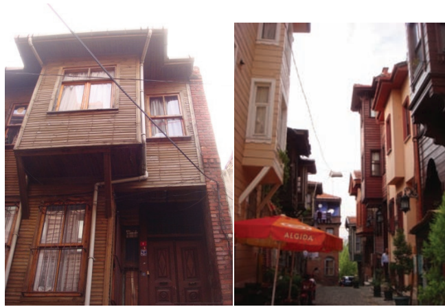
Figure 28 Listed timber buildings in a good condition
