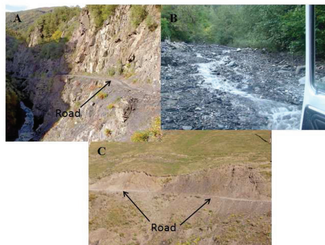
Figure 6.7: Hotspots examples of: (A) Rockfall; (B) Stream crossing road; (C) Landslide.
