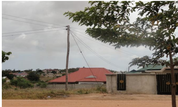
a) Buildings connected with electricity-Mivumoni
