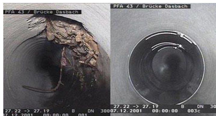
Figure 4: Sewer pipe point repair using a mechanical seal. Source: (Rausch, n.d.)
