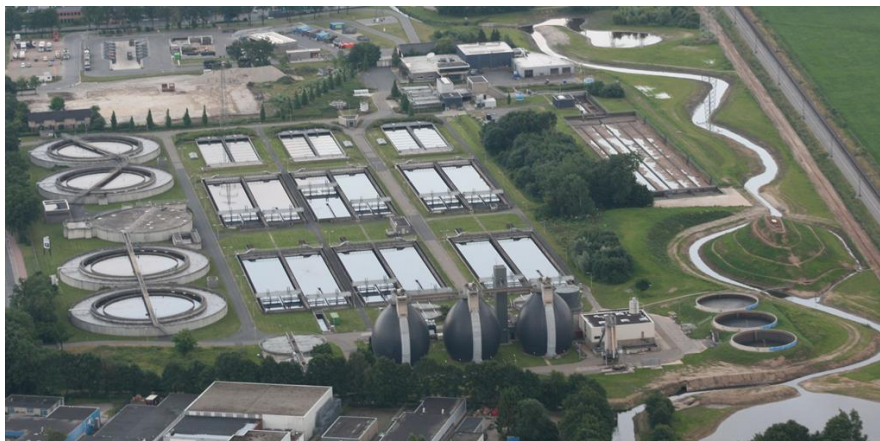
Figure 2.1.1: Wastewater treatment plant in Hengelo (Vechtstromen, 2013).
