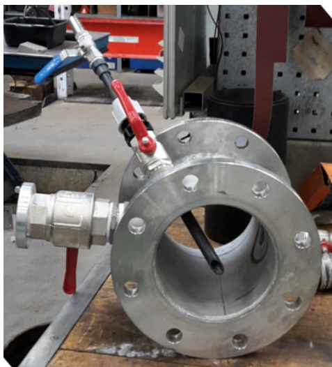
(a) Sampling point build in behind the venturi.
