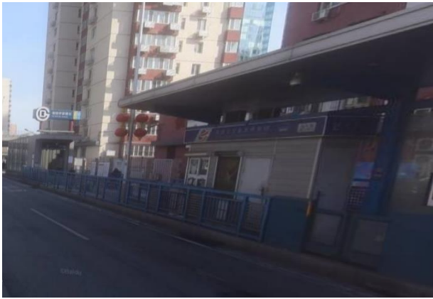
Figure 16 The exit is connected to the BRT station
