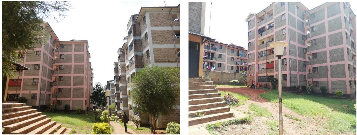
Figure 11: Housing units at the upgraded site. Source: Rahma fieldwork,(2020).
