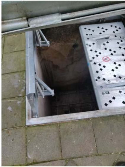
(a) Partly opened safety floor
