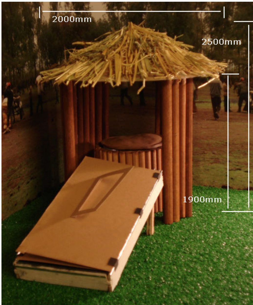
Illustration H.22: Measurements of hut around the baking plate
