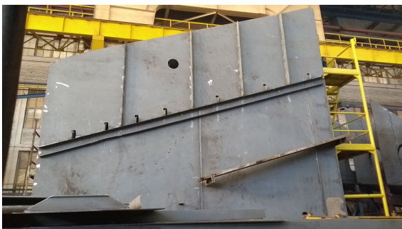
Figure 3.8: Vertical Assembly finished
