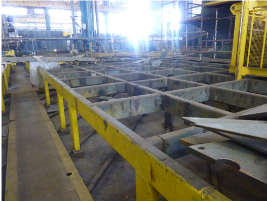
Figure 3.4: Building bed in Galati
