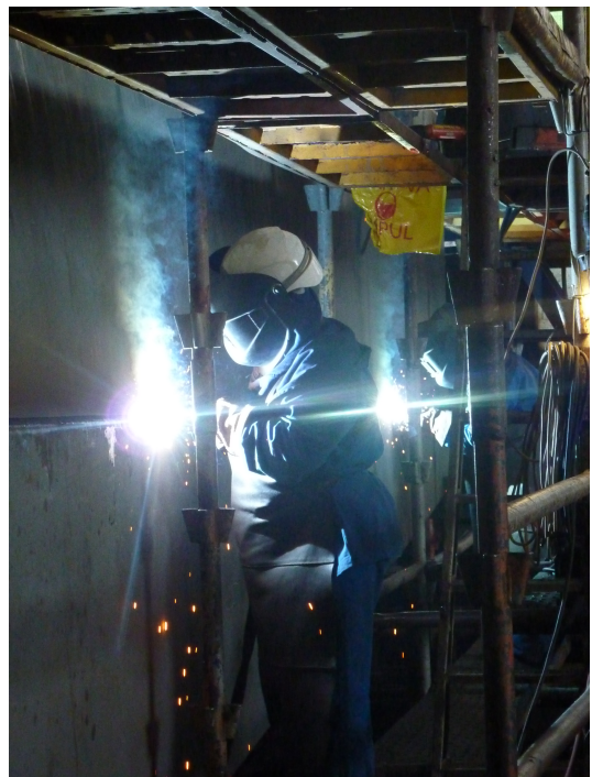
Figure 3.9: Final shell welding
