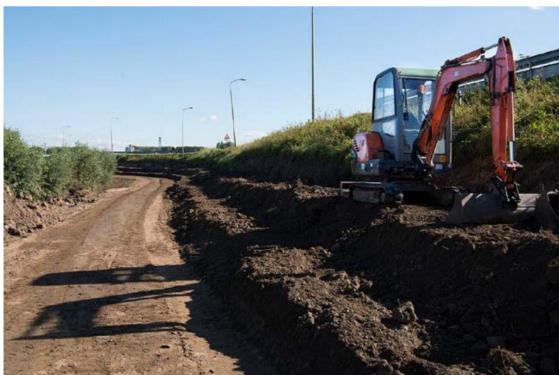
Figure 14: Applying a stair wise profile on the slope
