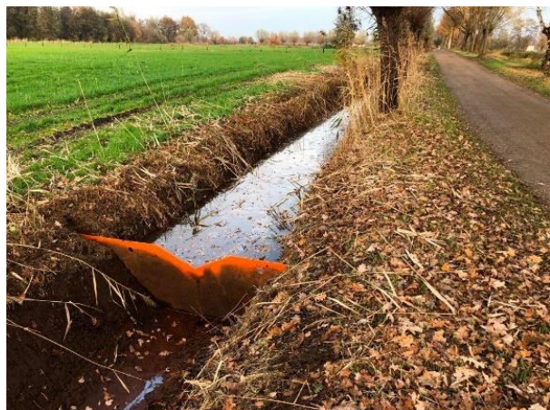
Figure 9: Road plate weir (Maas)
