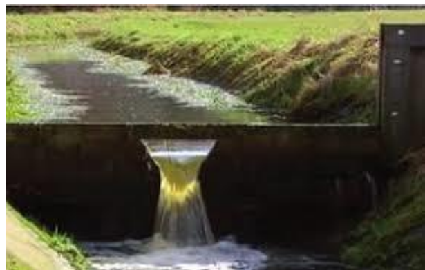
Figure 8: Pinch weir (VLM)
