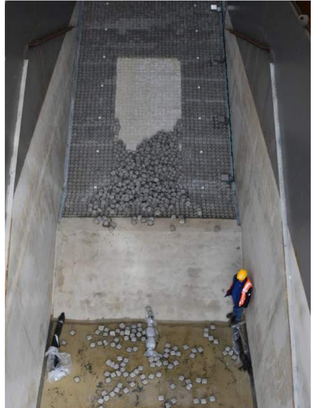
(b) Damage on the Grassblocks after Test03.
