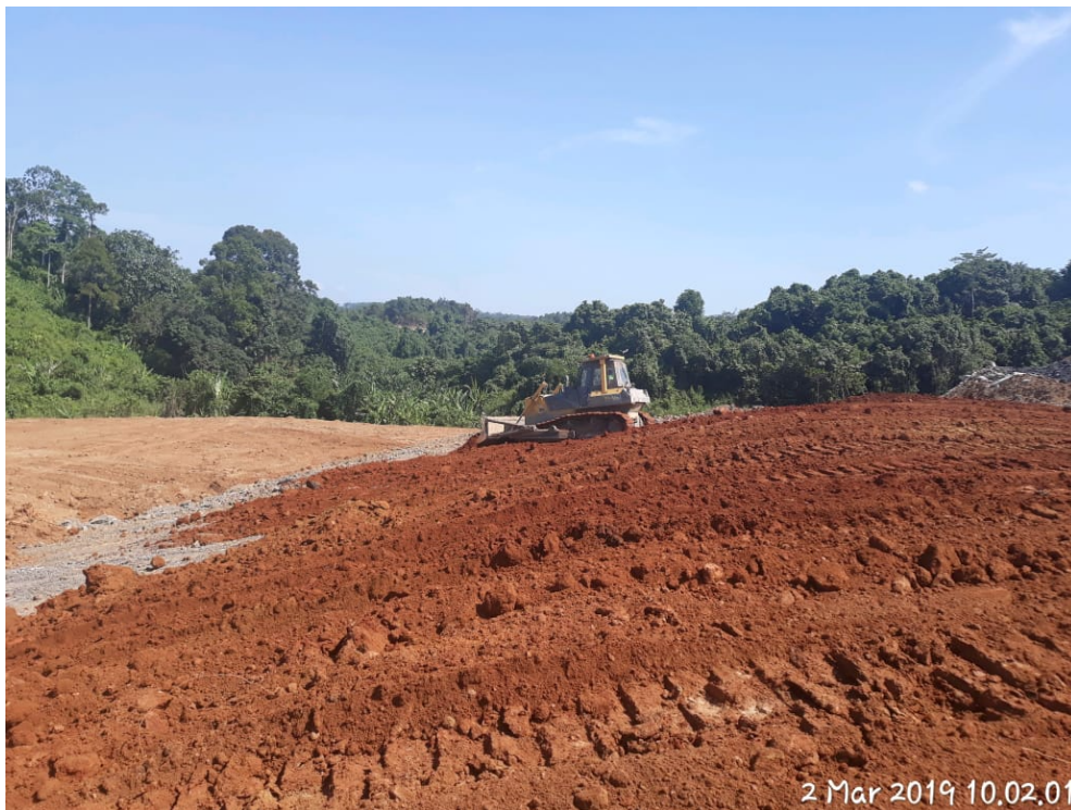
Figure 6. Topsoil Spreading
