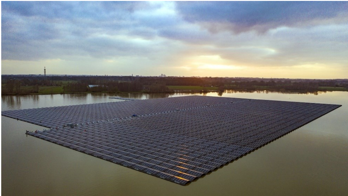
Figure 1: Floating PV system in Bomhofsplass, Zwolle, sized 27 MWp (BayWa, 2020).
