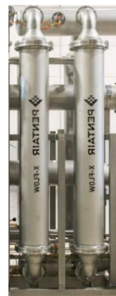
Figure 10: Membrane modules BMF S4 (source: Pentair)
