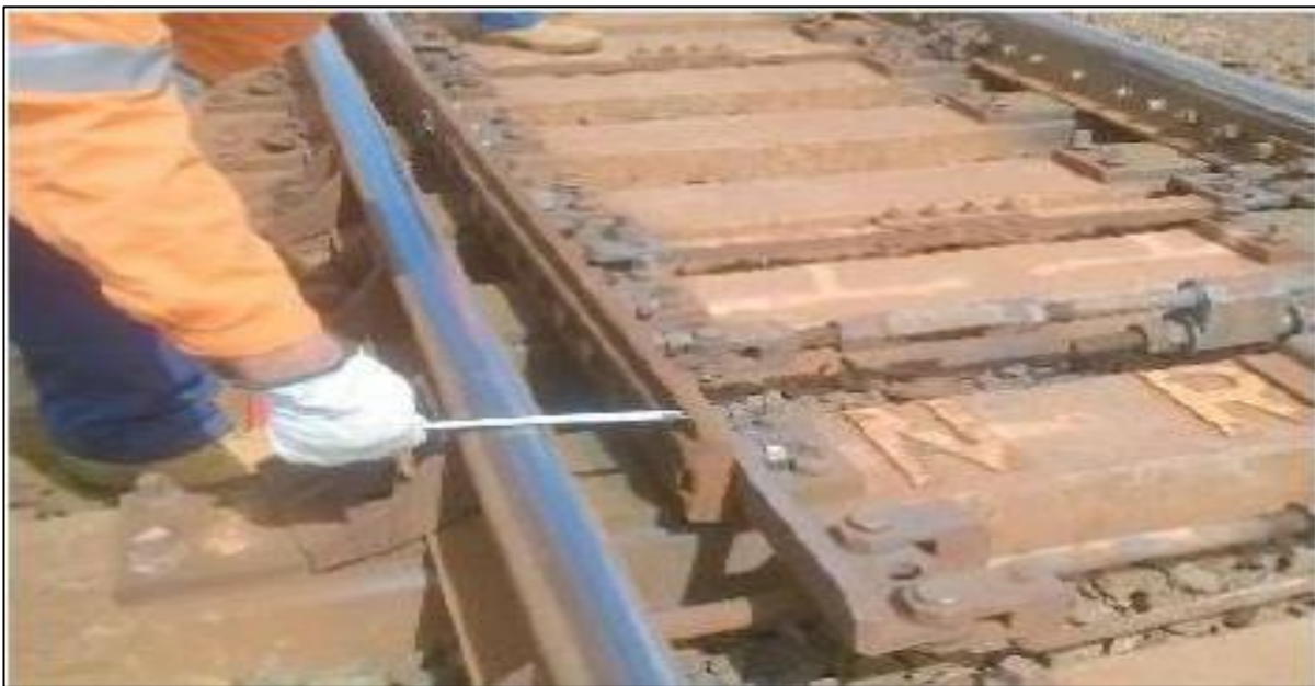
Figure 1-3 An operator measuring the distance between the stock rail and its switch rail manually. This is a manual measurement in contrast to what is done in this work from a point cloud (Source: Fugro Raildata).
