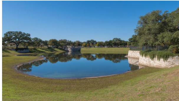
Figure 33 - Example of a retention pond (Presley, 2019)
