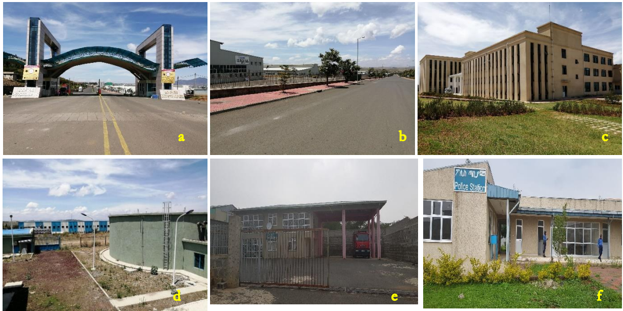
Figure 21: (a-f) Infrastructure supply in Bole Lemi I Industrial Park (Source: Yisehak fieldwork, 2021)
