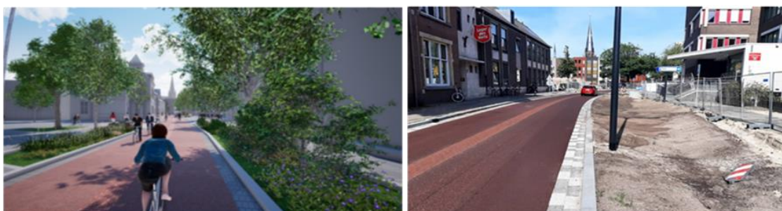
Figure 3-4 Image of the visualization (left) and in construction (right) of the Molens straat with cycle street with wadi and green on the side
