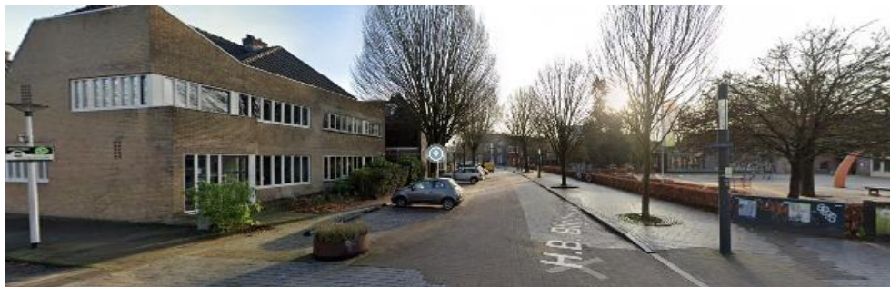
Figure 3-3 Images of the street H. B. Blijndensteinlaan that is mostly flooded
