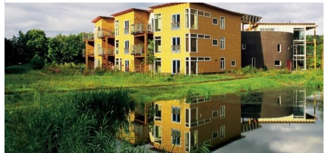
Figure 2-14 Image of Rainwater pond
