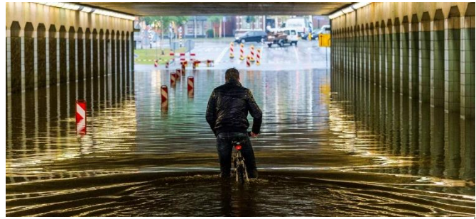
Figure 2-1 Flooded Princess tunnel near the station of Enschede Source: Wouter Borre, 2019
