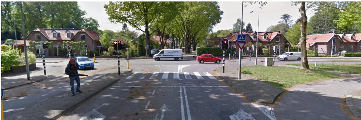
Figure 8.4: Traffic lights at the Eikenlaan accessing Klinkenbergerweg (Google, 2021)
