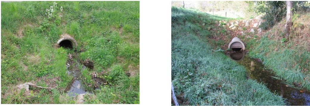
Figure 2: An example of a culvert (left) and a pinch culvert (right) (Hehenkamp, M. , 2019)
