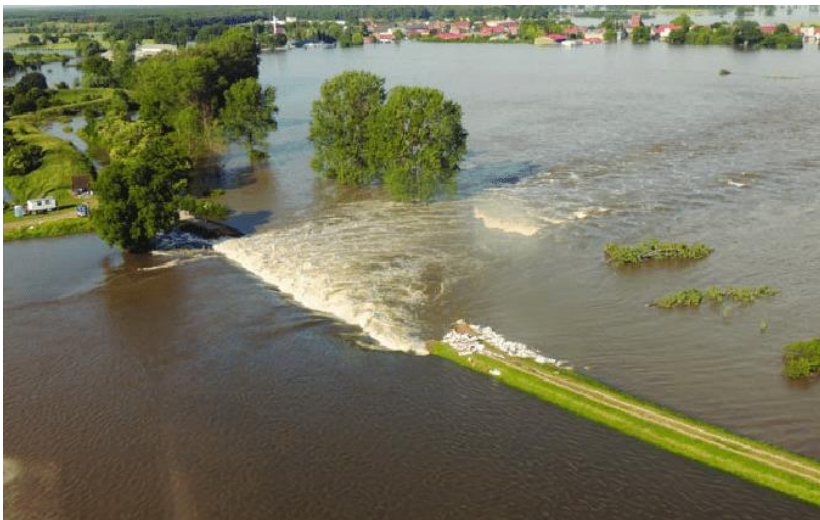
Figure 1 – The flooding of the hinterland caused by a dike breach. Note: reprinted from Jüpner (2018).
