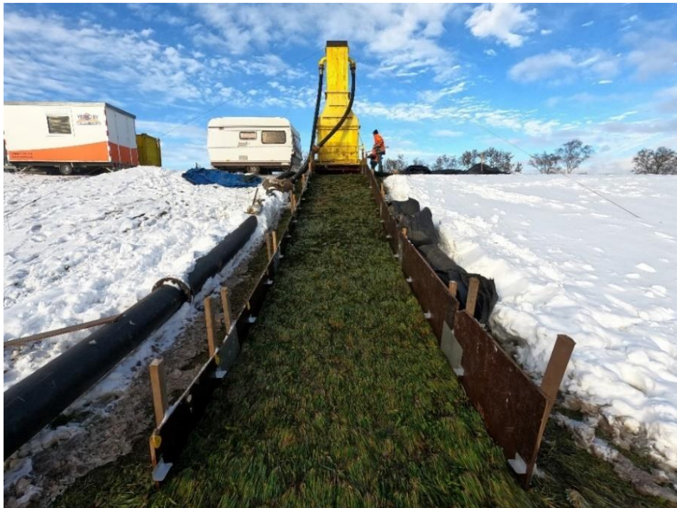
Figure 11 – The wave run-up simulator set-up for test section 2 at test location one at the Vecht dike. The wave run-up simulator was developed by Van der Meer Consulting B.V. and Infram. Note: reprinted from Mom et al. (2021)
