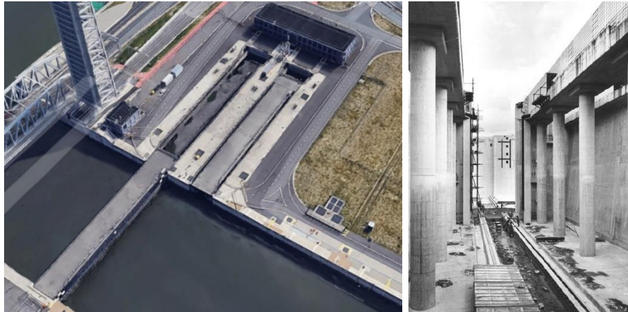
Figure 1. Kieldrecht lock with a closed and open gate respectively (left) [5], gate chamber of a rolling gate in the marine lock in Terneuzen (right) [3].
