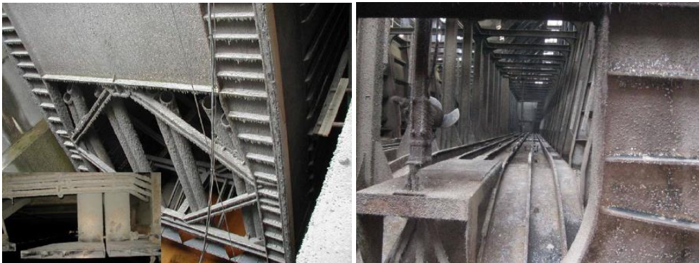
Figure 6. Venturi system inlet detail (left) [6] and Internal gate structure and mixer for debris and sediment control (right).
