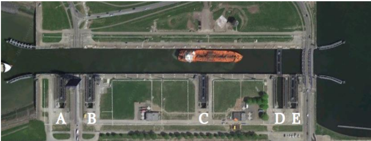
Figure 8. West lock Terneuzen [18].
