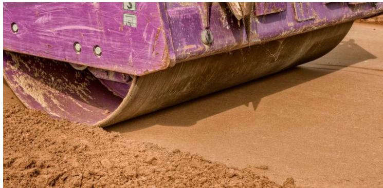
Figure 2: Trisoplast being applied by a heavy roller (Trisoplast Mineral Liners, 2021)
