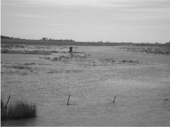
*Figure 48: Upstream view over Alfonso bridge during a low risk flood (February 2010). It shows the limnigraph station, the backwater effect that had been foreseen by HECRAS and the large inundation plain that will be inundated in case of extreme flooding. Reducing the peak to Pergamino*
