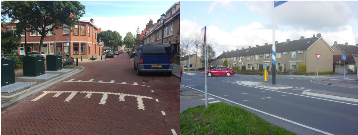
FIGURE 6: A) STREET WITH A PAVEMENT STONE SURFACE (MAKE BV, CIVIELTECHNISCH ADVIESBUREAU, SD), B) A STREET WITH AN ASPHALT SURFACE (DE BAAN, SD)
