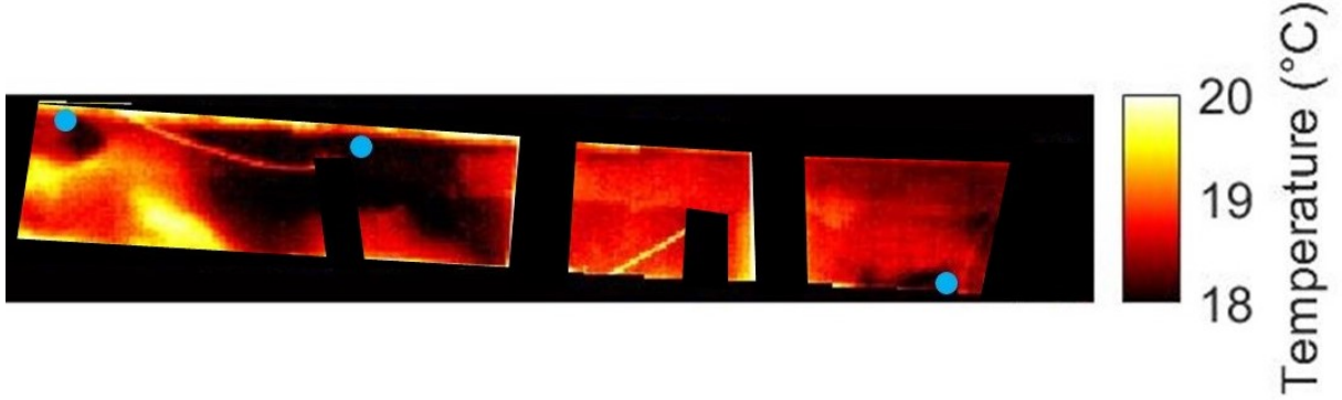
Figure 5.6: The locations of the three seepage spots in the remaining data set, indicated with a blue dot. The seepage spot in the middle is active during the whole data set, the seepage spots on the left and on the right are not active during the complete data set. The obstacles as shown in Figure 5.1 are kept out of the analysis.
