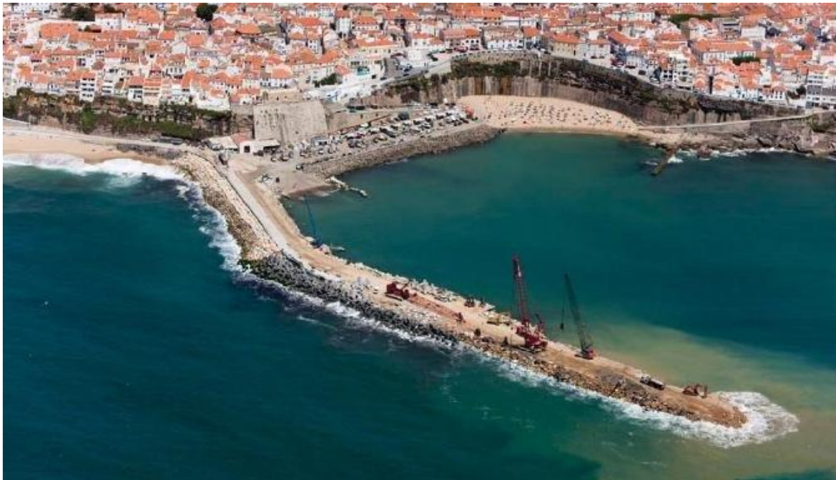
Figure 1: Reconstruction of the breakwater of the port of Ericeira (Henriques et al., 2014).
