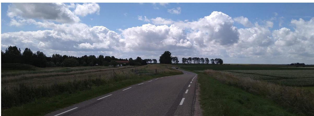
Figure 8 – Compartmentalizing dike, with compartment 1 on the right side, and compartment 2 on the left side. Location photograph shown in Appendix 3.
